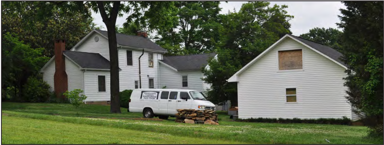
Figure 44. Magnolia Vale, West Side with Garage
