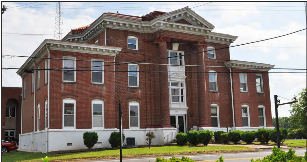
Figure 69. Rockingham County Courthouse, Front, North Side
