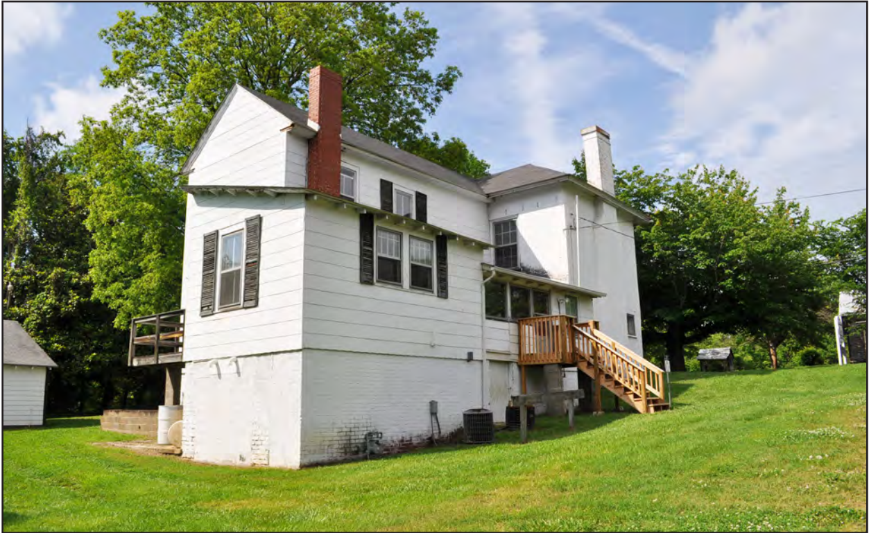
Figure 112. Martin-Irving House, South and East Sides
