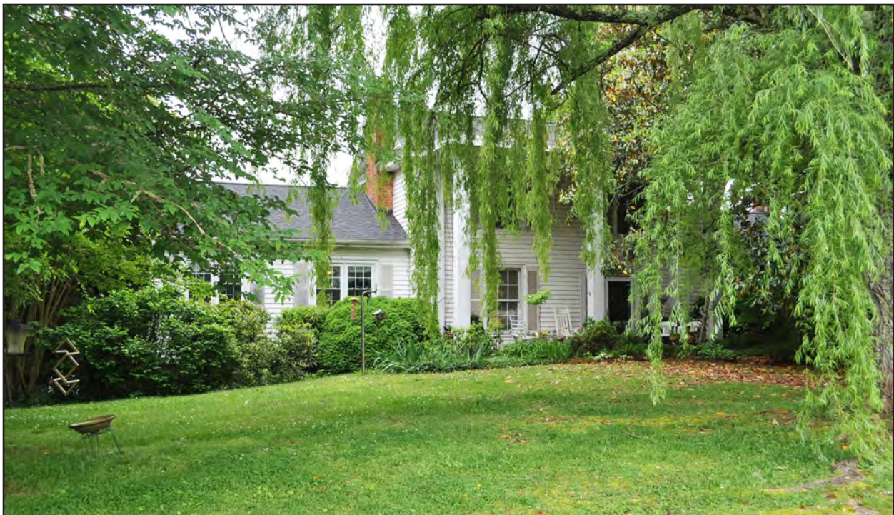
Figure 43. Magnolia Vale, Front, North Side
