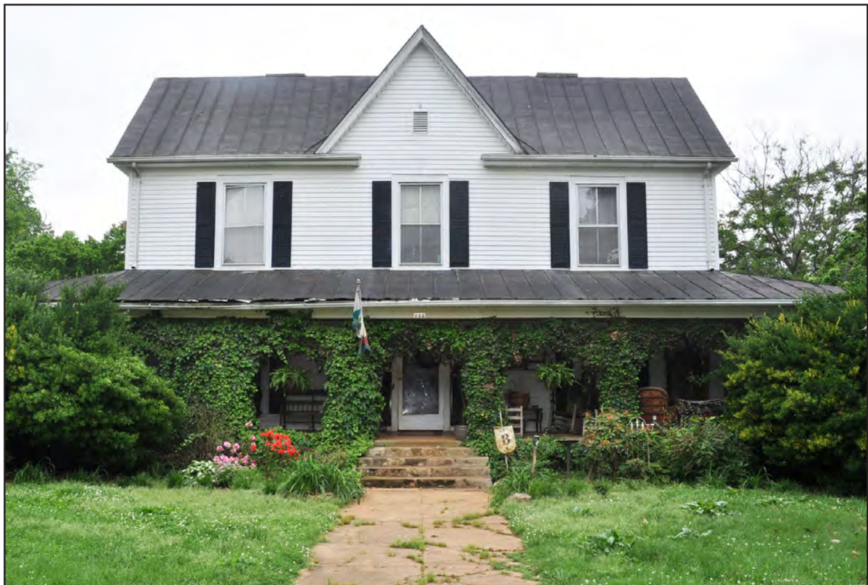
Figure 22. James Thomas Smith House, Front, North Side
