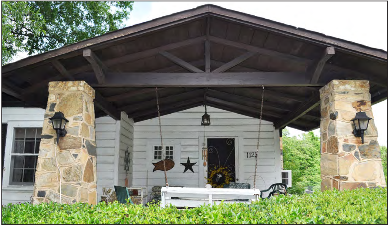
Figure 102. Mitchell-Adams-Perdue House (#1), Porch Detail
