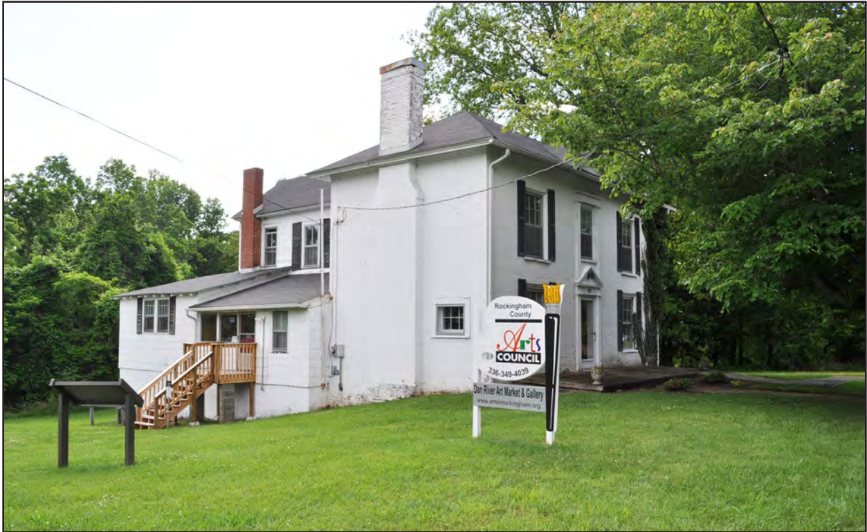
Figure 110. Martin-Irving House, East and North Sides
