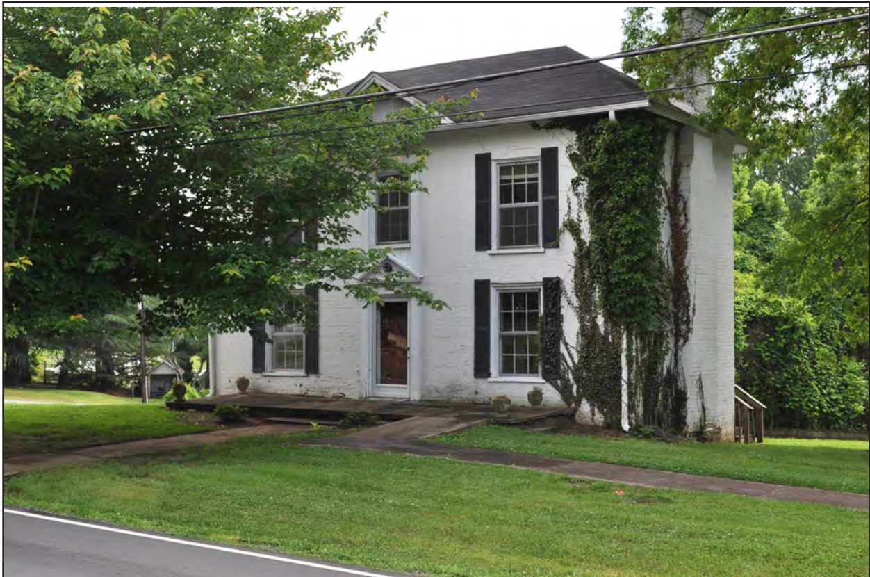
Figure 106. Martin-Irving House, Front, North Side
