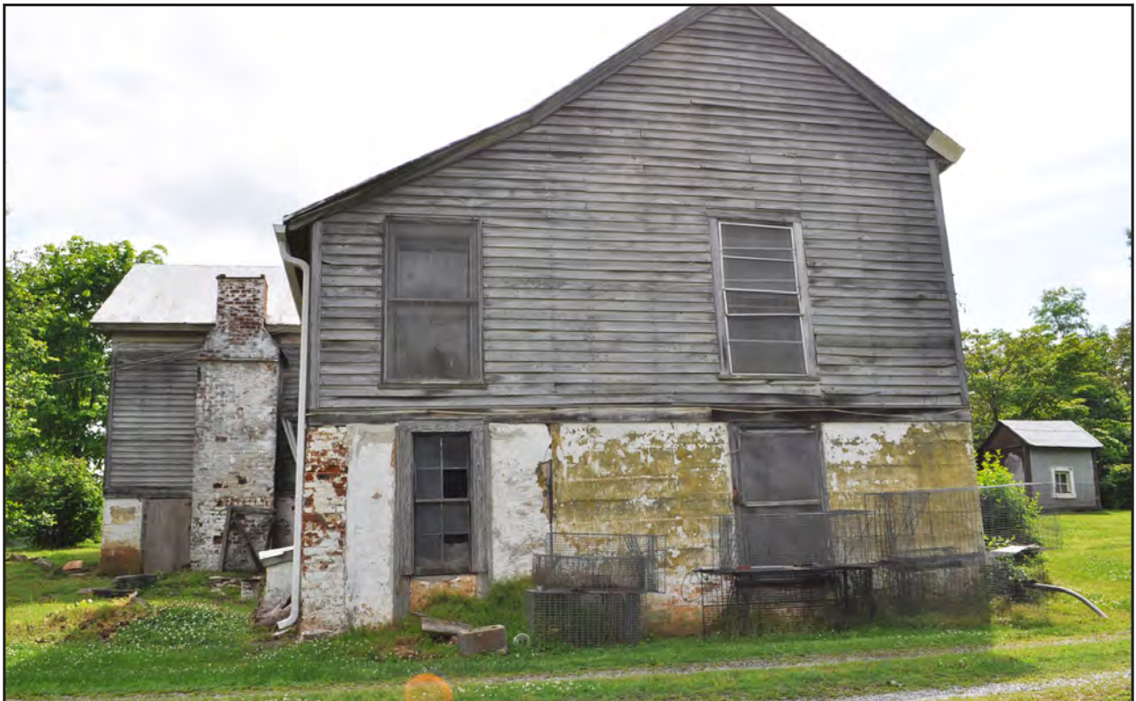
Figure 96. R.G. Mitchell House, East and North Side of Ell
