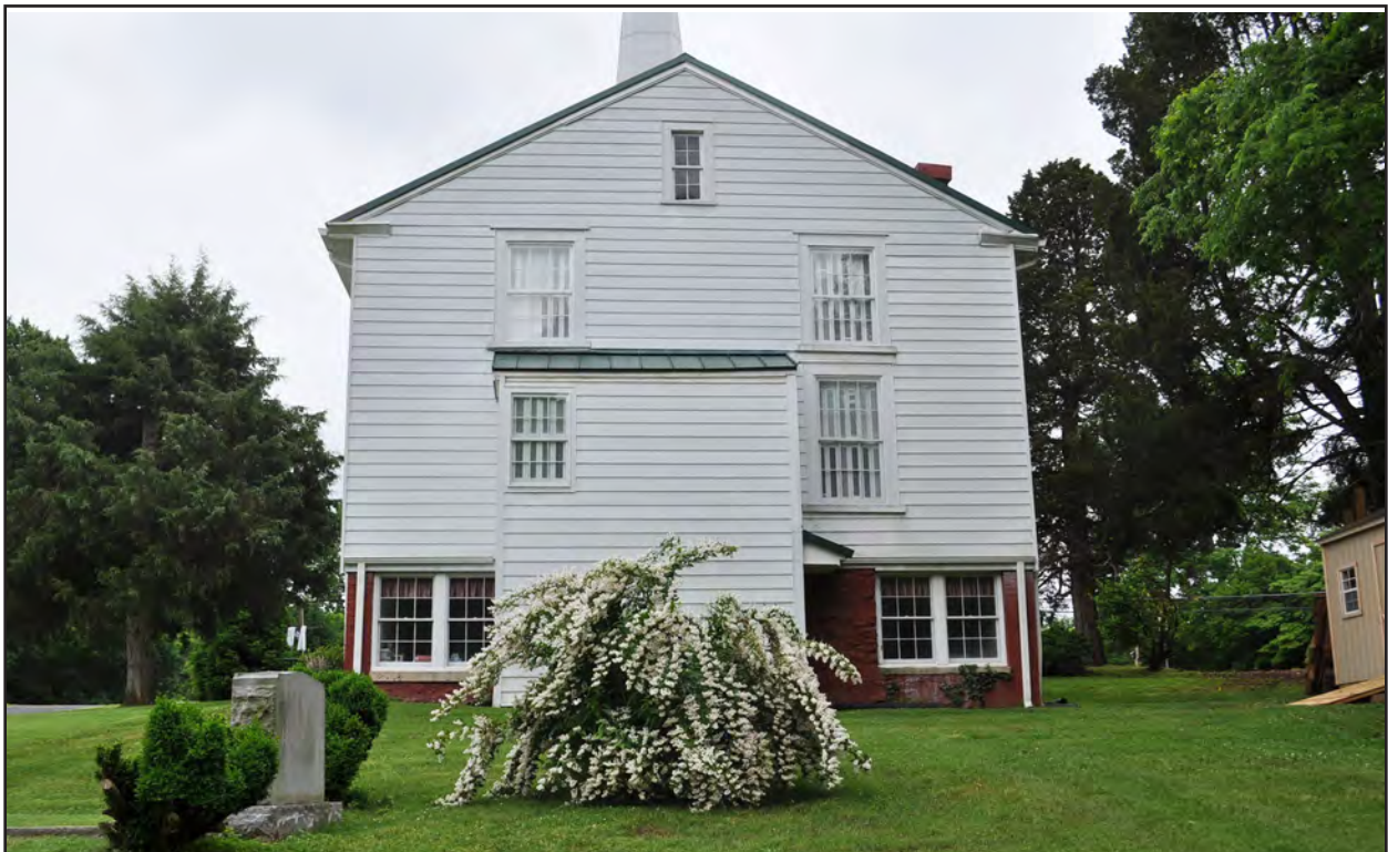
Figure 33. Wentworth Presbyterian Church, North Side
