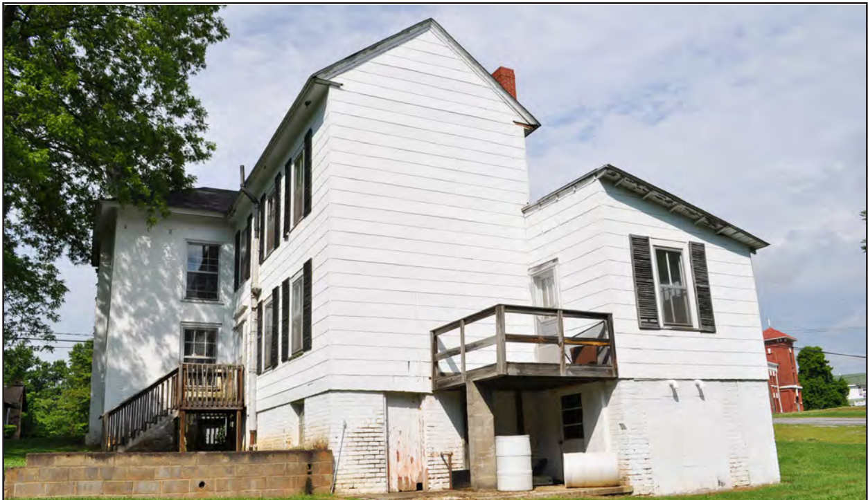
Figure 111. Martin-Irving House, South Side
