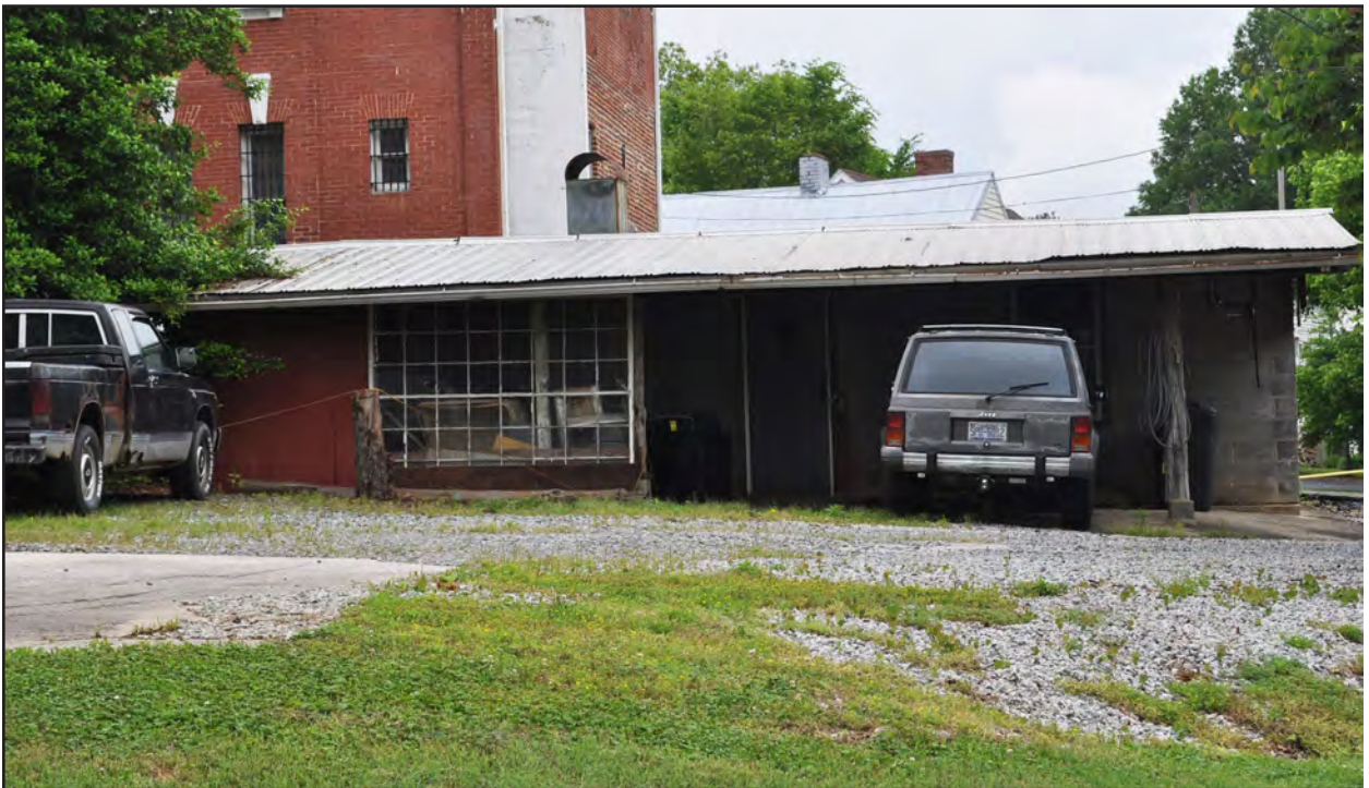
Figure 68. Thomas A. Ratliffe Store, Storage Shed, East Side
