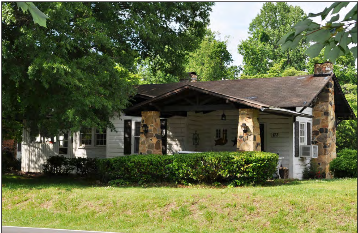
Figure 99. Mitchell-Adams-Perdue House (#1), Front (South) and East Sides
