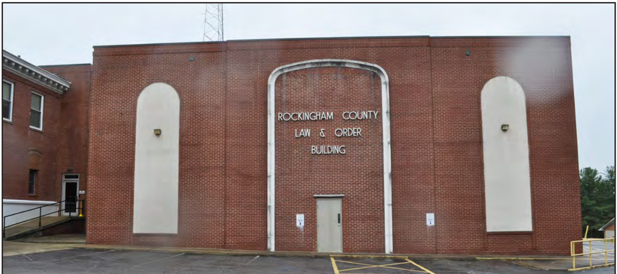
Figure 75. Rockingham County Courthouse, Law and Order Building, Front, North, Side
