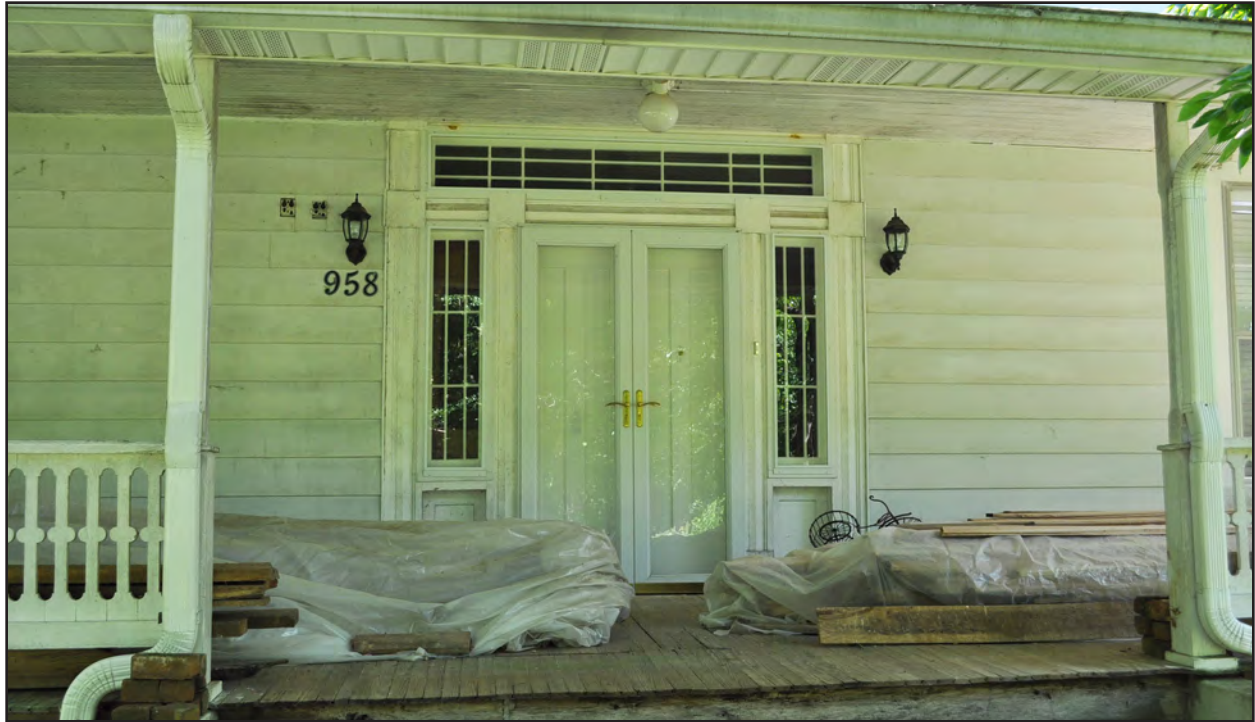
Figure 16. Alfred M. Scales House, Entry Detail
