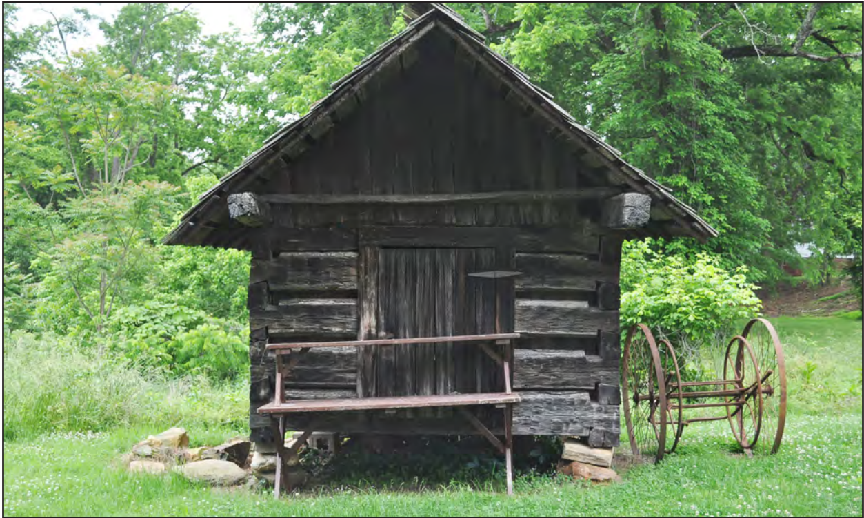
Figure 62. Wright Tavern Outbuilding, Crib, West Side
