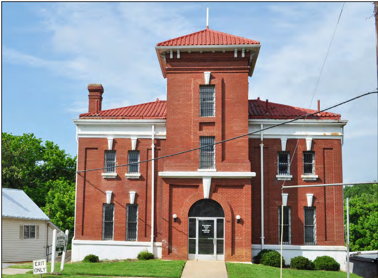
Figure 76. Rockingham County Jail, Front, South Side
