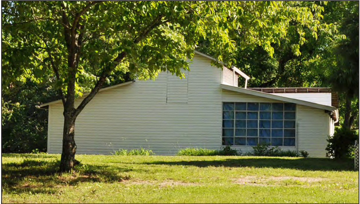
Figure 20. Detail of the Alfred M. Scales House Outbuildings, Gabled Shed
