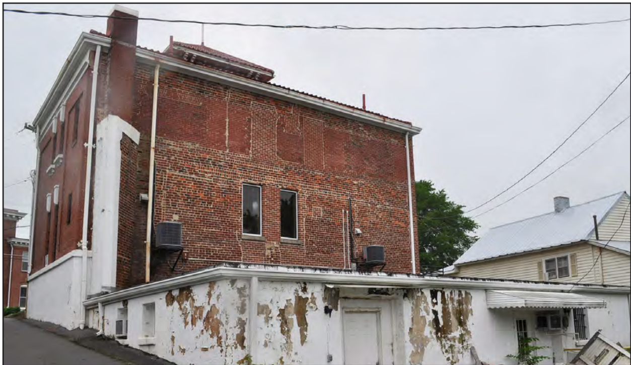
Figure 80. Rockingham County Jail, Rockingham County Jail, North and East Sides
