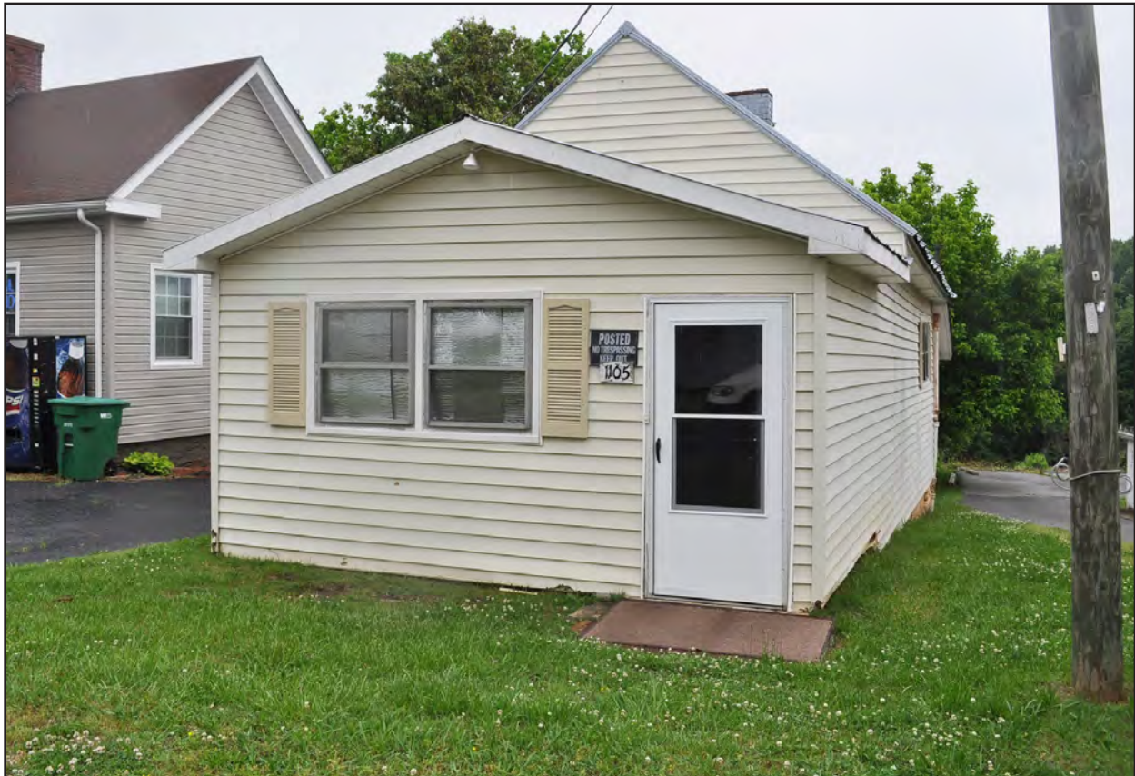
Figure 83. McMichael Law Office, Front, South Side
