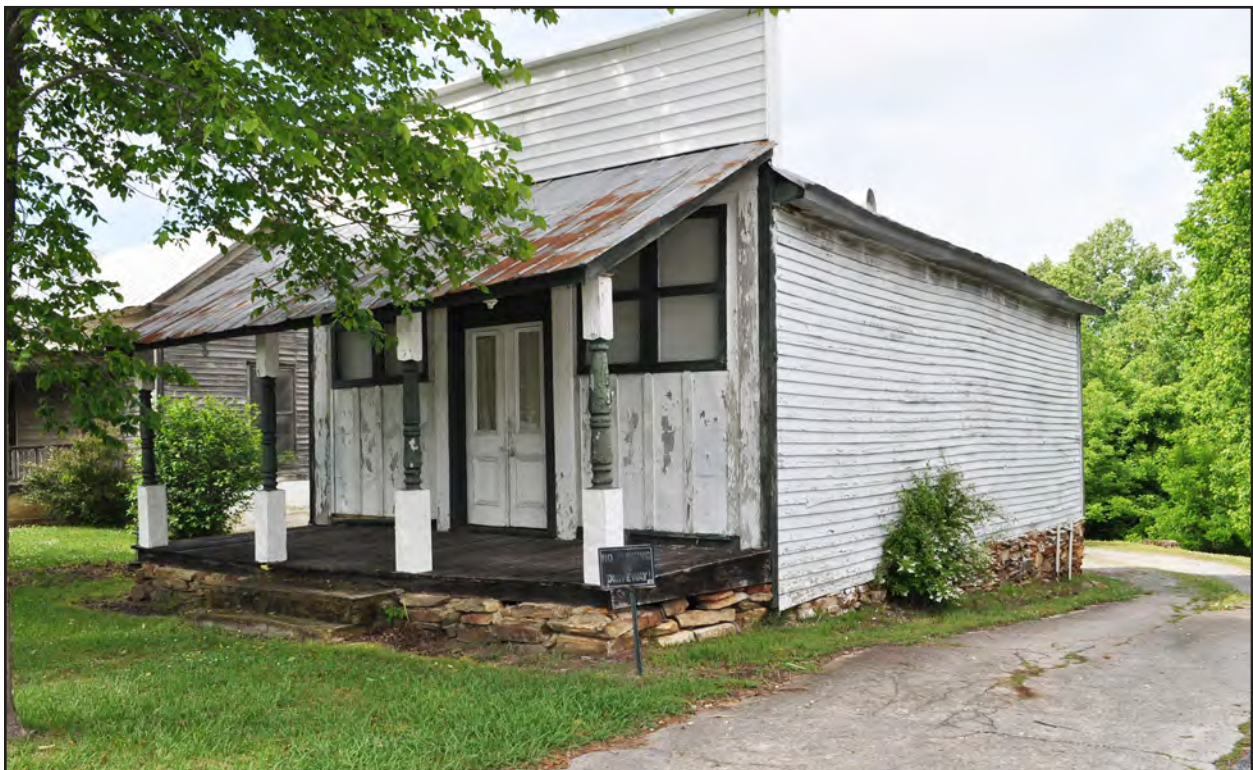
Figure 87. R.G. Mitchell Store, Front (South) and East Sides
