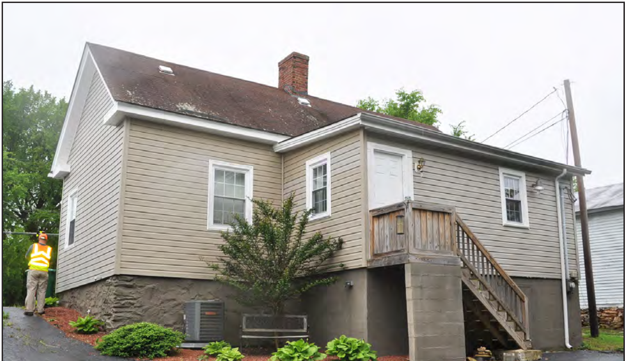
Figure 86. Scott-Reid Law Office, North and East Sides
