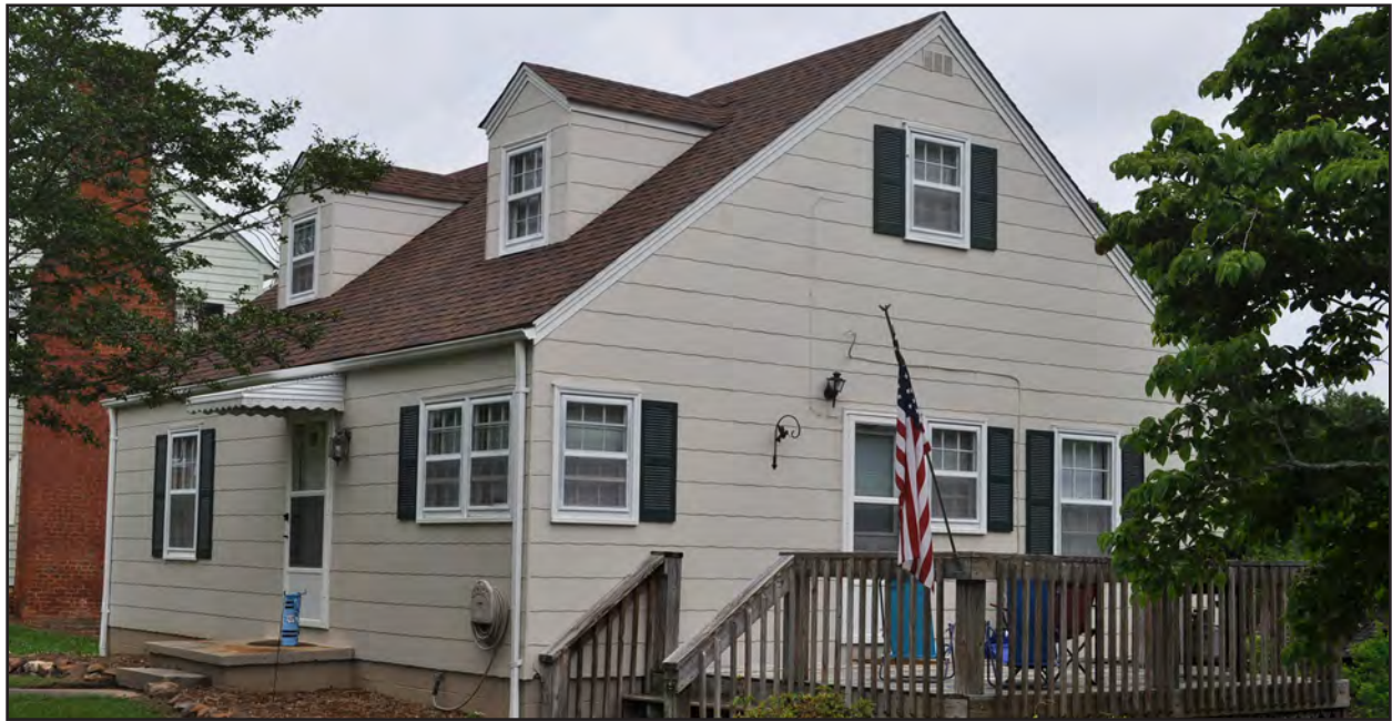
Figure 49. Wentworth Presbyterian Church Manse, North and East Sides
