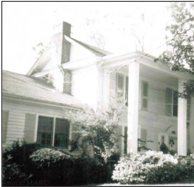
Figure 45. Historic View of Magnolia Vale, Front, North Side
