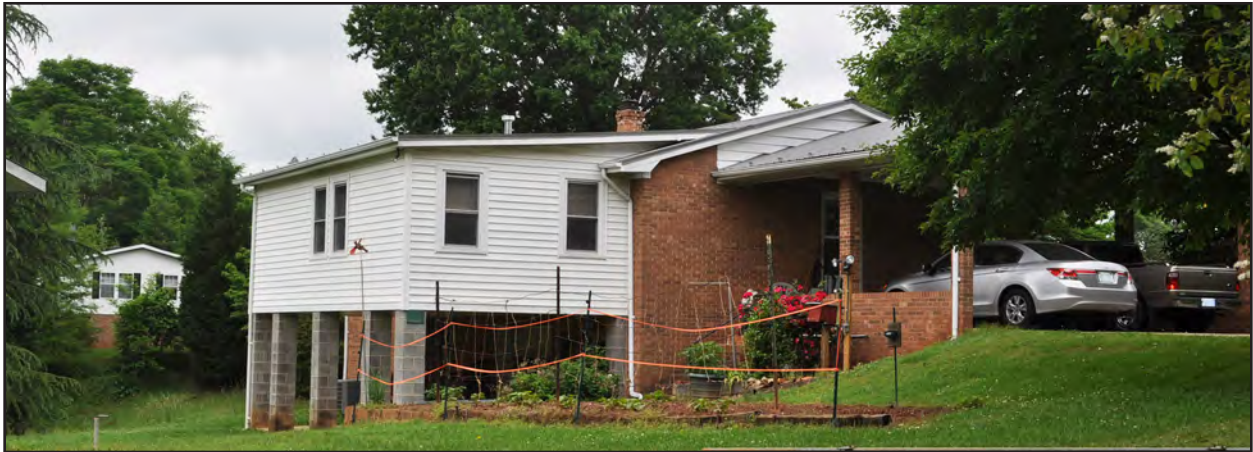
Figure 28. Parlier House Outbuildings, Metal Shed and Carport
