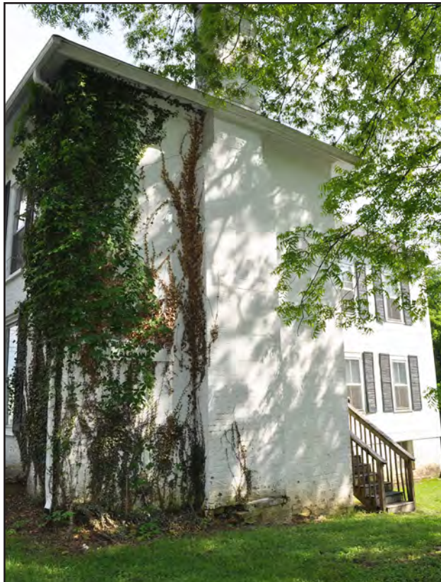
Figure 108. Martin-Irving House, Stepped-Shoulder Chimney, West Side
