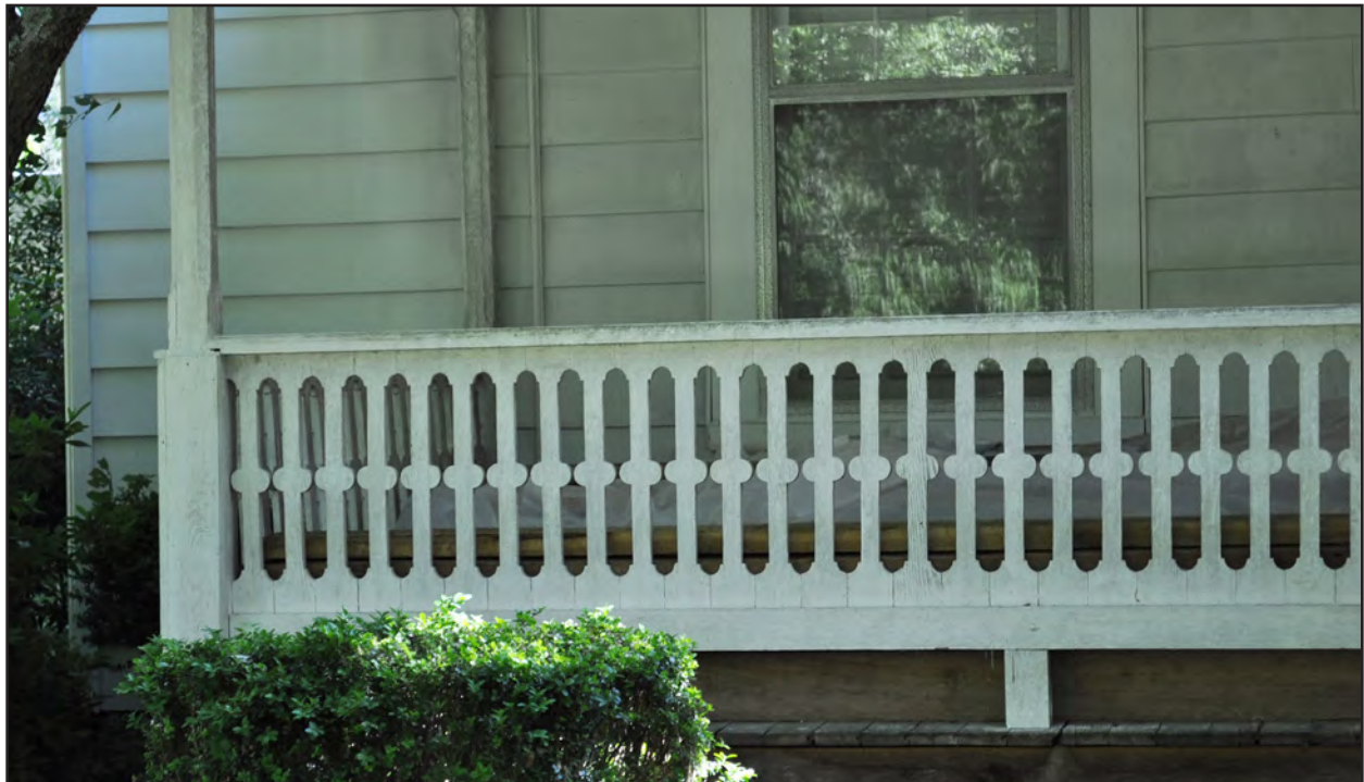
Figure 17. Alfred M. Scales House, Porch Balustrade Detail
