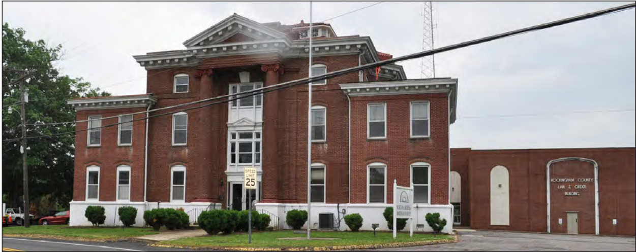
Figure 71. Rockingham County Courthouse, Cupola Detail
