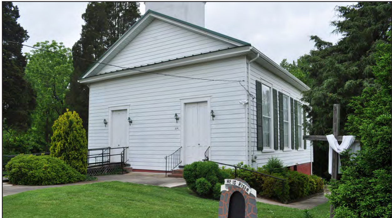
Figure 31. Wentworth Presbyterian Church, South and East Sides
